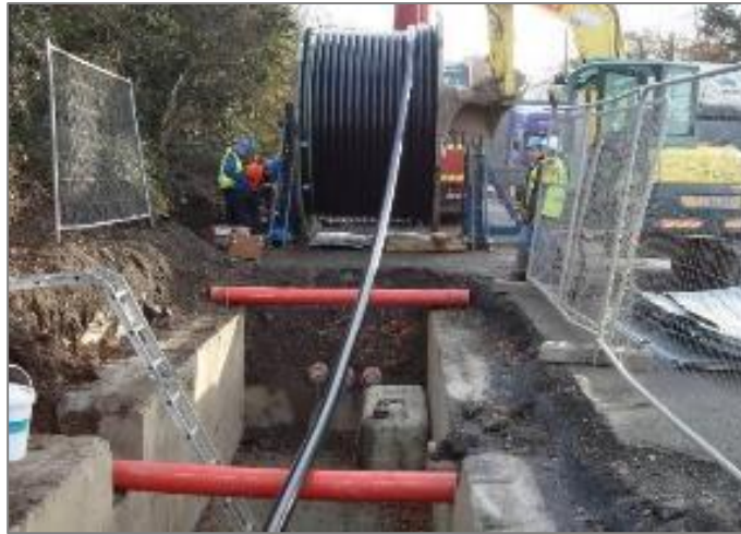
Figure 16: HV cable pulling procedure (Standard drum set-up)
