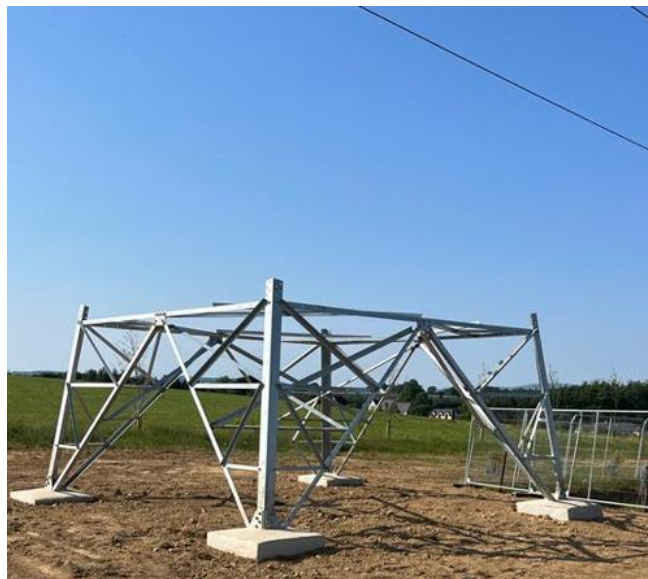
Figure 5: Base of mast structure backfilled
