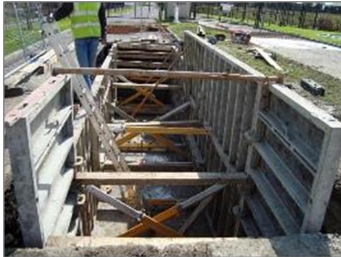
Figure 14: Standard joint bay under construction (in-situ)
