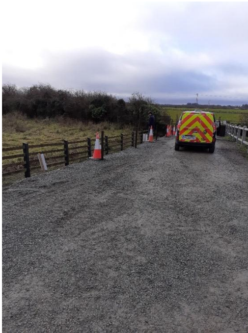
Figure 21: Crushed Rock Roadway
