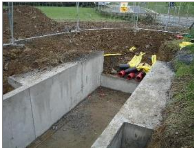
Figure 15: Example of completed joint bay prior to cable installation (in-situ)
