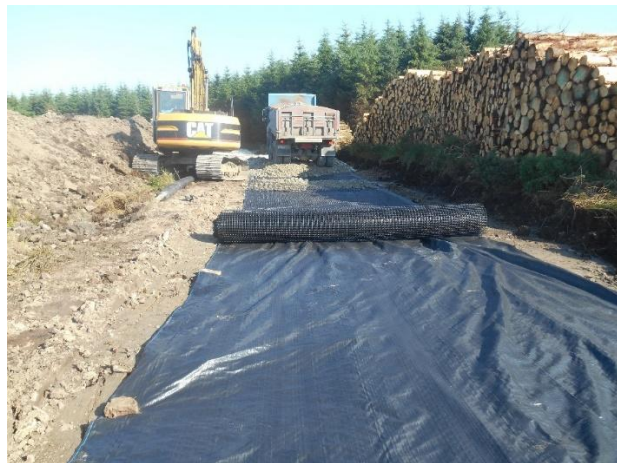
Figure 22: Crushed Rock Roadway Build-up With Geotextile
