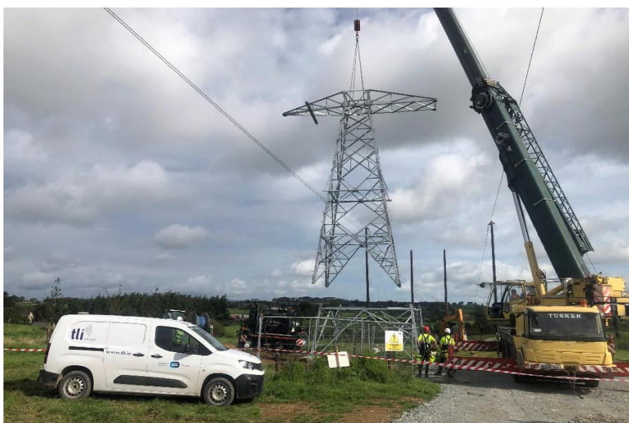
Figure 23: Crane pad and laydown areas.
