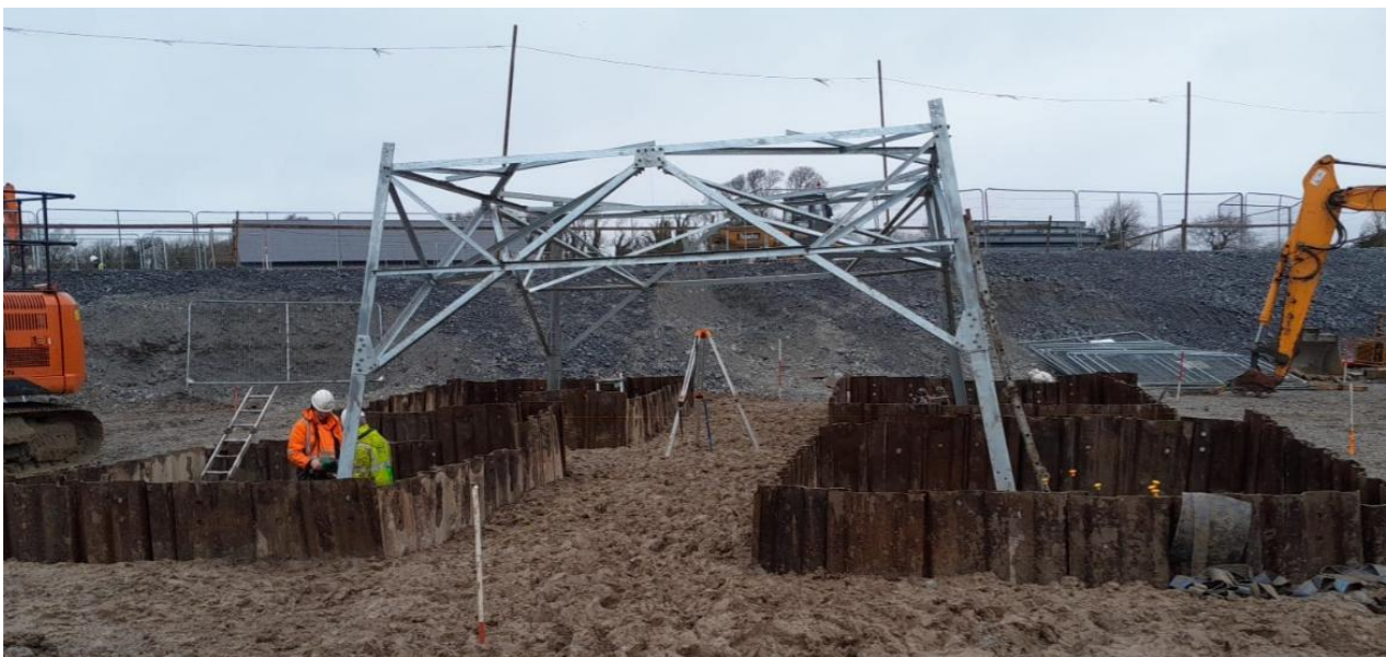
Figure 3: Sheet Piled Foundations
