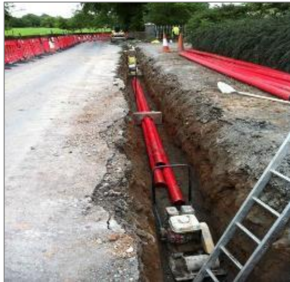
Figure 9: Typical 110kV Underground Duct Installation
